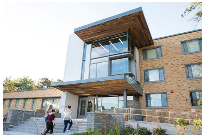
A newly renovated Waterbury Hall reopened in August 2015.
