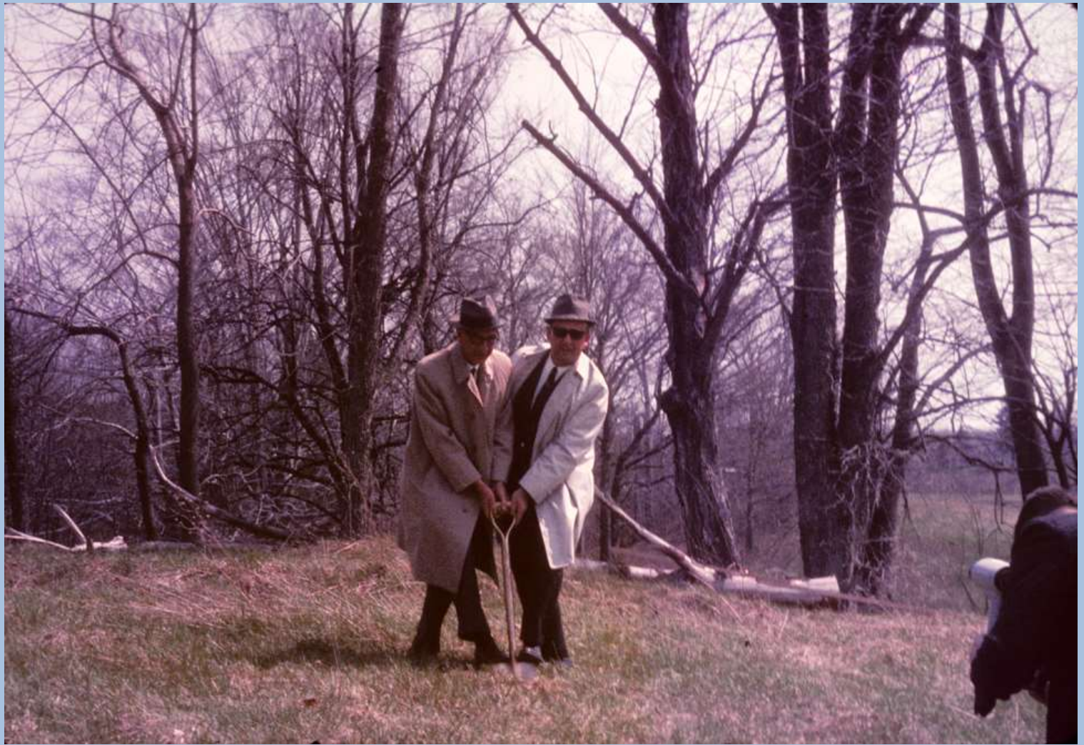
Ground breaking for building May 1966. Slide is labeled Bud Coward (may be Foster Brown) and Sam Costaldo.
