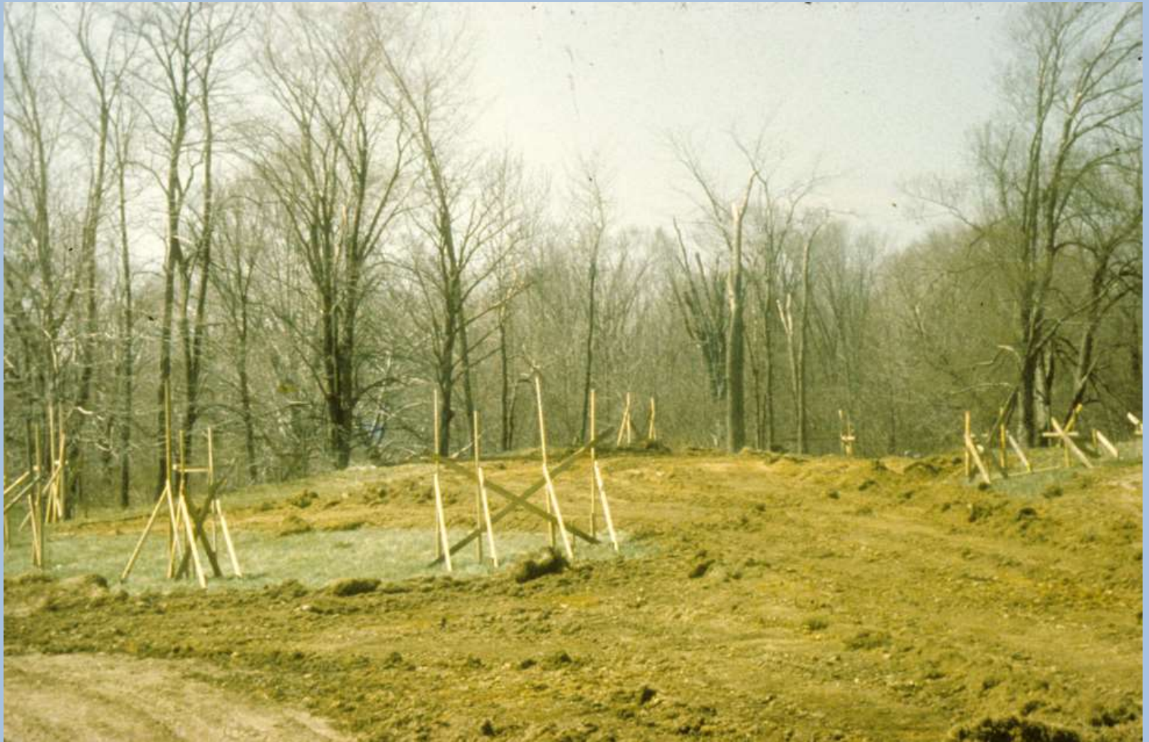
Grading markers for lab building 1966.
