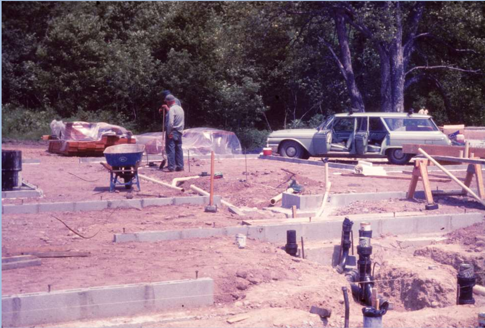
Foundation construction for lab building 1966 looking east or south east.
