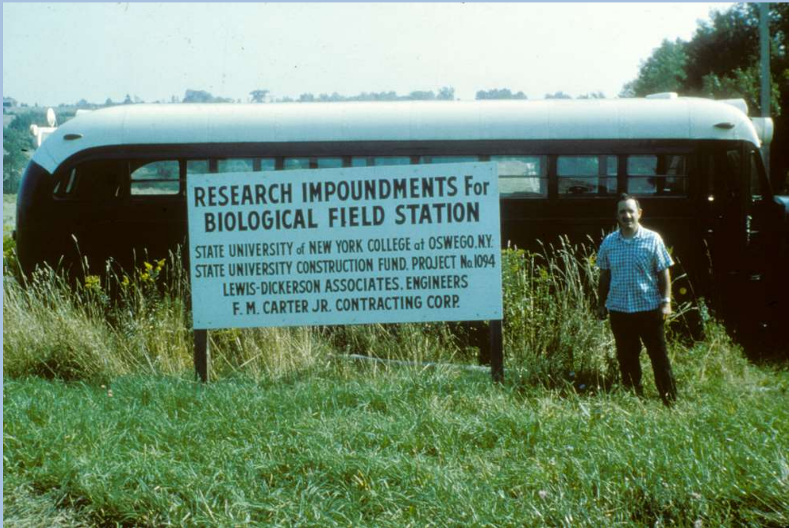
Floyd M. Carter headquarter trailer set up near intersection of Cemetery and Brownell Roads. John Weeks early-1960s.
