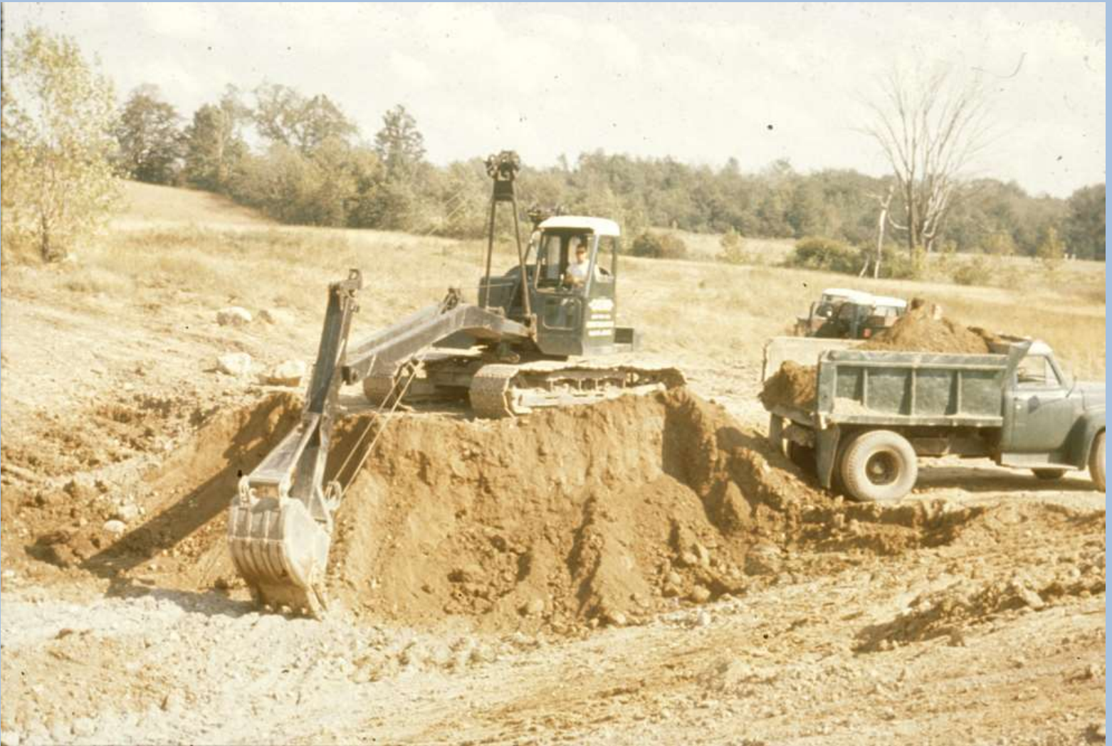
Digging canal to “fish ladder” backhoe sits on original ground level. Truck is close to canal level.
