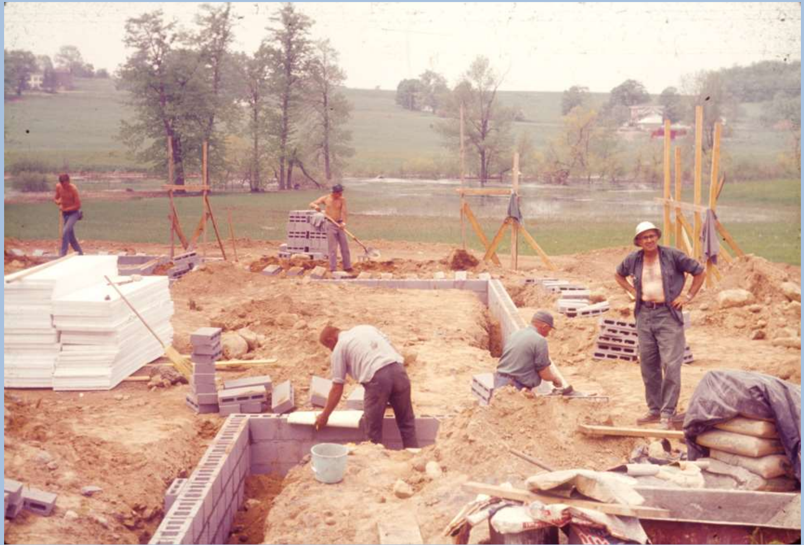
Foundation work 1966. Looking westward across pond to Cemetery Road.
