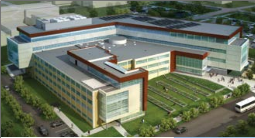
Top: Artist's view of the Richard S. Shineman Center for Science, Engineering and Innovation, looking east.
