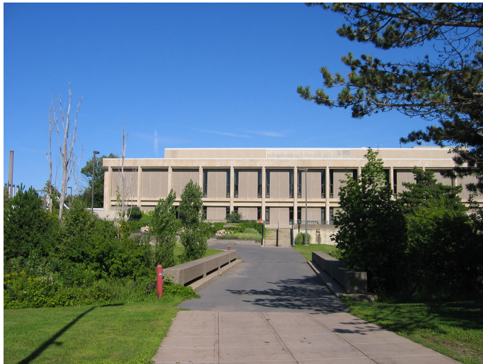
Tyler Renovation will Provide New Opportunities for Connection to West Campus Housing
