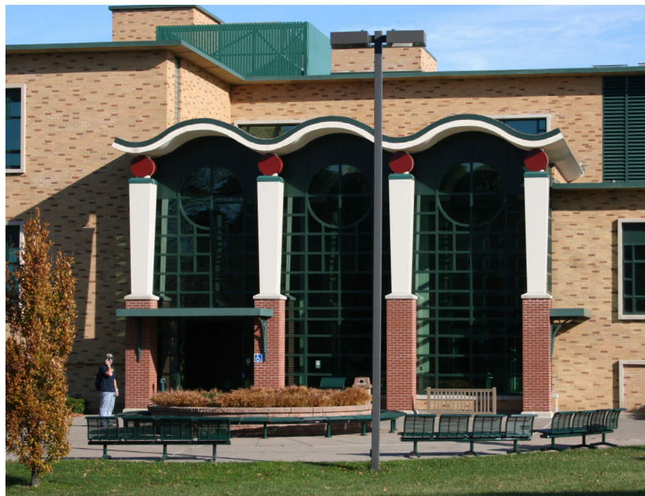
New Entry to Rich Hall
