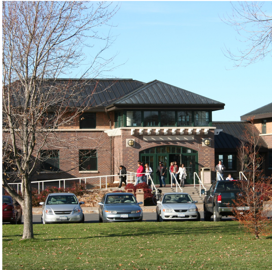
Renovation and Addition to Johnson Hall
