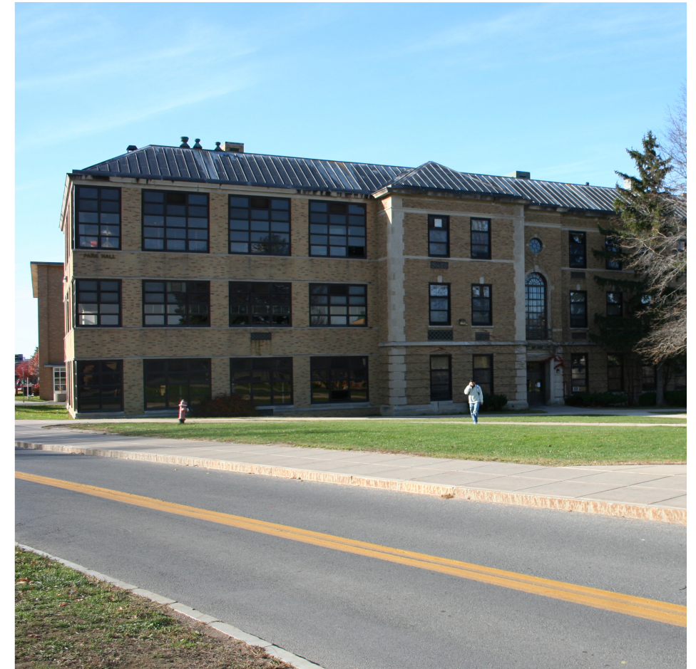
Addition to Park Hall
