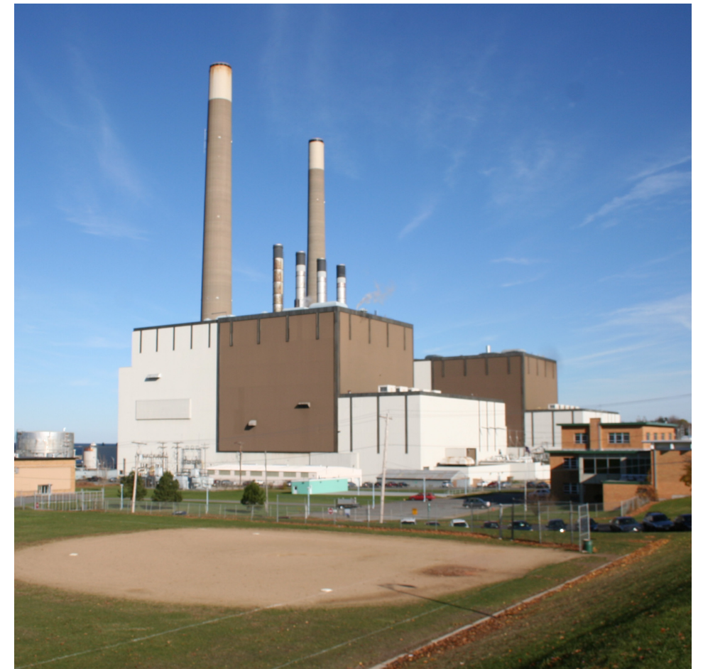
Power Plant Next to Campus
