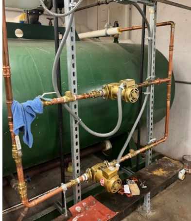
Picture 16: Gas Service with a Regulator
