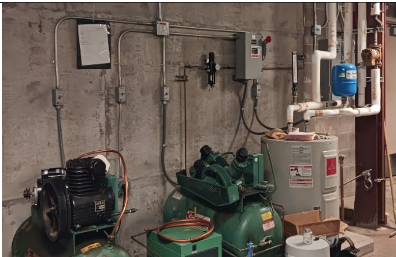
Picture 7: Air Compressors
