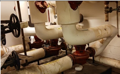
Picture 3: Condensate Receiver Unit
