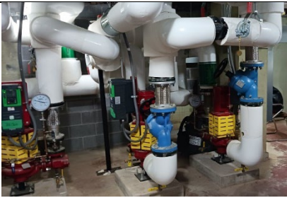
Picture 2: Hot Water Pumps
