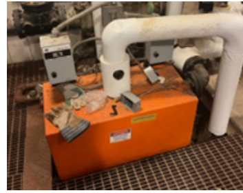
Oneida duplex condensate receiver
