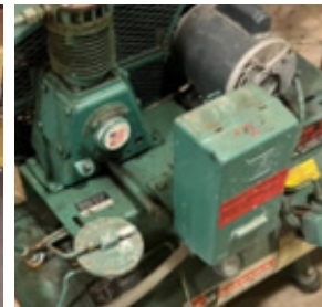
Oneida compressor for pneumatic controls
