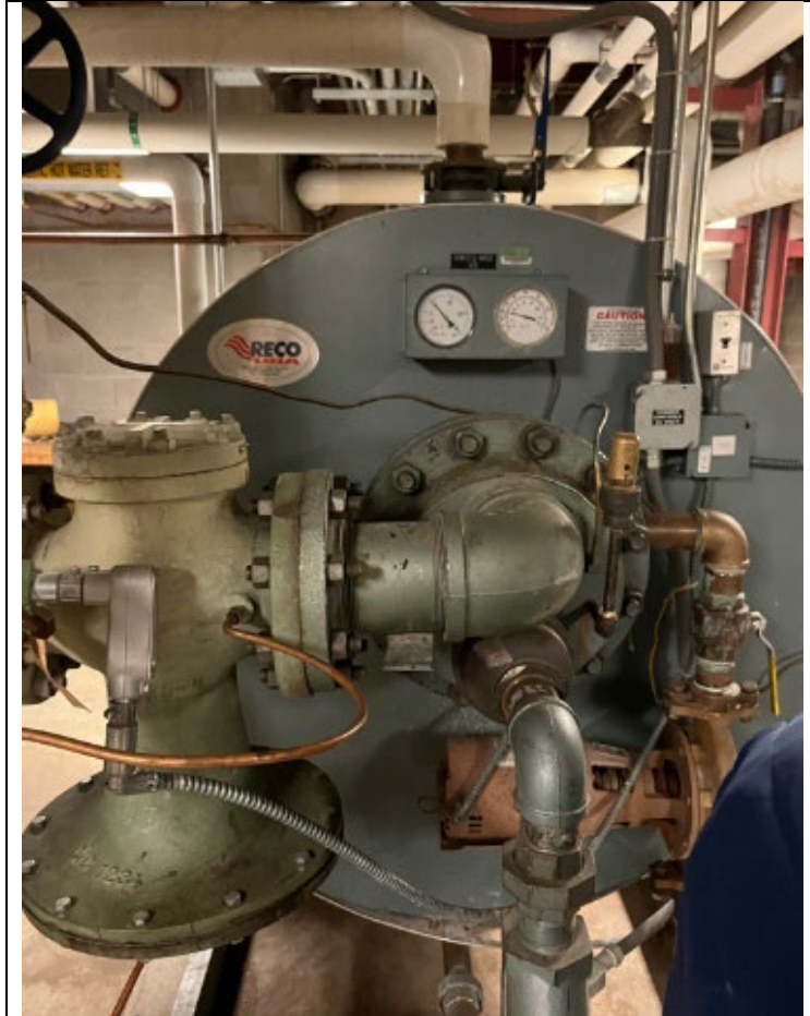
Picture 15: Domestic HW Tank
