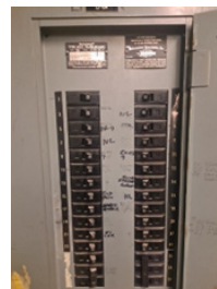
Aging Westinghouse panel in Hart.
