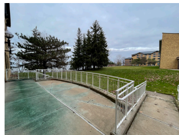
Riggs Hall patio surface requires cleaning. Railings need to be repainted.
