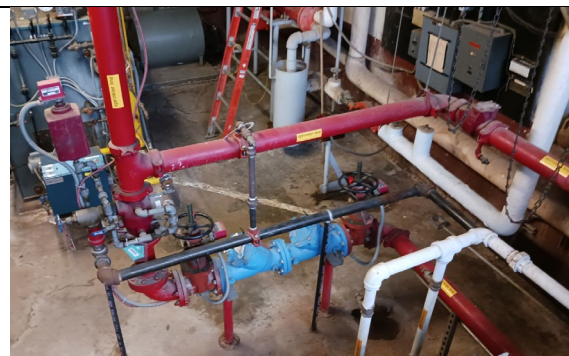
Picture 15: Fire sprinkler BFP and Alarm Check Valve
