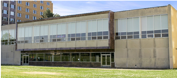
Cladding at Cooper DH shows signs of moisture infiltration.
