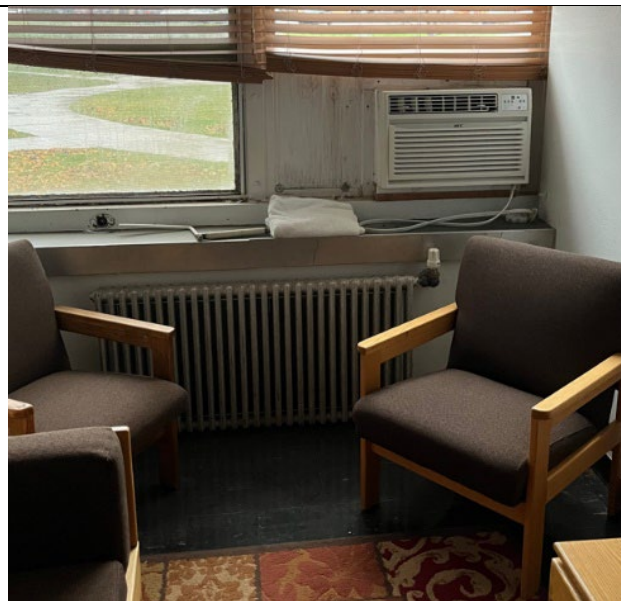
Picture 5: Radiator and Window AC unit
