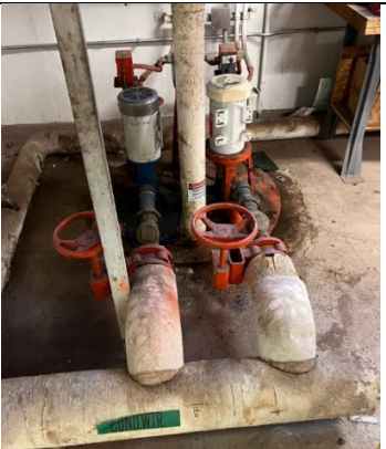
Picture 3: Condensate Receiver Unit
