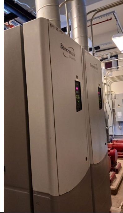
Picture 1: Heating Boilers
