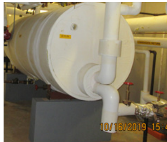
Seneca domestic hot water storage tank
