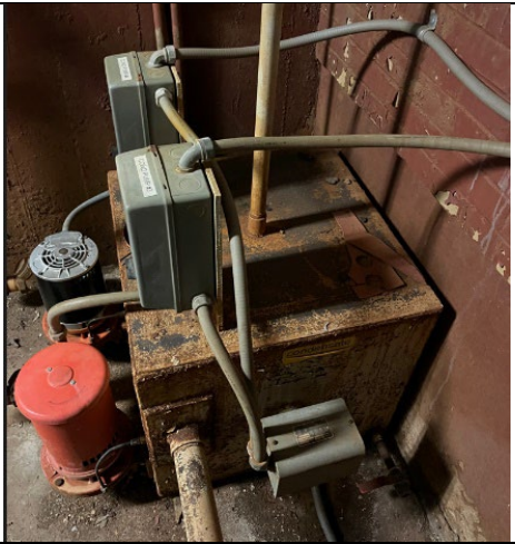
Picture 4: Condensate Receiver
