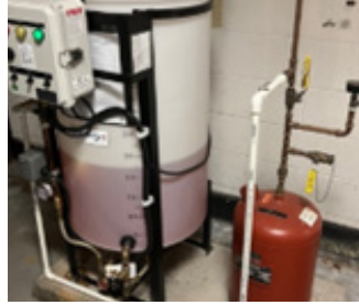
Cayuga glycol tank for chilled water system
