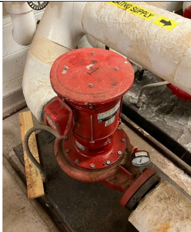
Picture 4: Hot Water Pump
