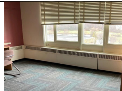
Picture 4: Hot Water Convectors
