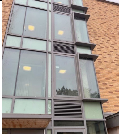
Picture 5: Corridor Exhaust Louvers
