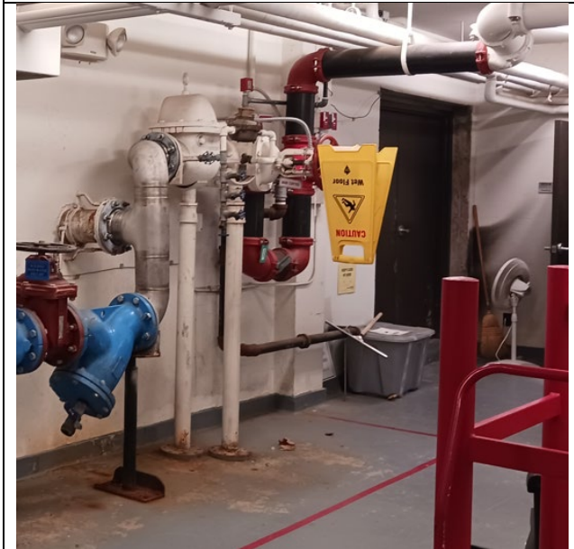
Picture 14: Combined domestic and fire water incoming service with a single check valve backflow preventer on the fire water side
