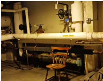
Onondaga water service and meter
