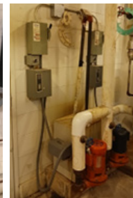
Duplex condensate receiver in Cooper
