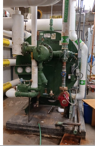
Picture 15: Steam-Fired DHW Heater
