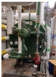
Steam-fired DHW, Waterbury. Similar unit in Scales.
