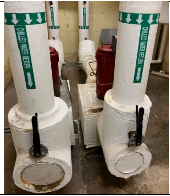
Picture 8: Primary Loop CHW Pumps
