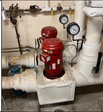
Picture 2: Hot Water Pumps
