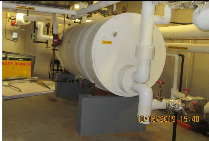
Picture 7: Domestic HW Tank
