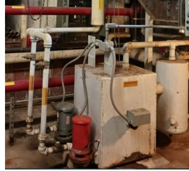
Picture 3: Condensate Receiver
