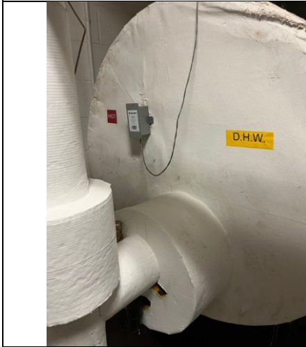
Picture 13: Domestic HW Tank
