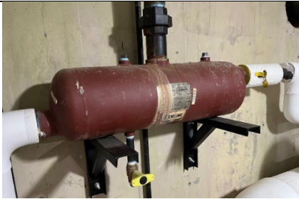
Picture 4: Heat Exchanger
