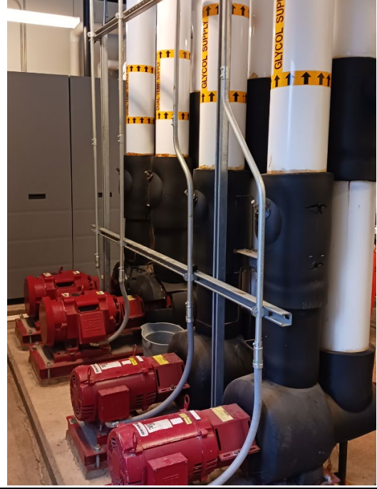
Picture 2: Heating and Cooling Pumps
