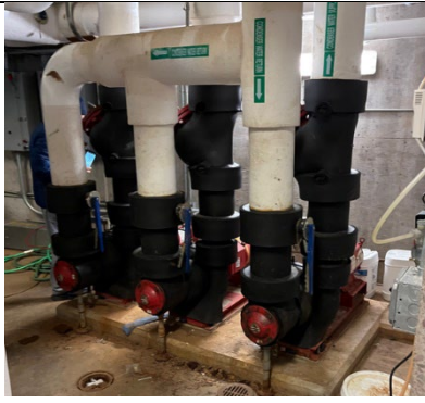
Picture 7: Condenser Water Pumps
