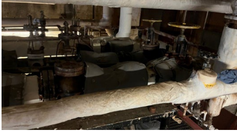
Picture 1: Pressure Reducing Valve Station
