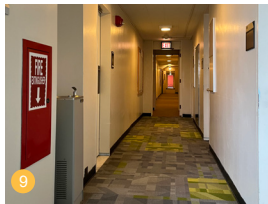
Knob hardware on student room doors and non-accessible water fountain on residence floor.
