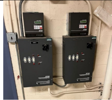
Picture 3: HW Pump VFDs
