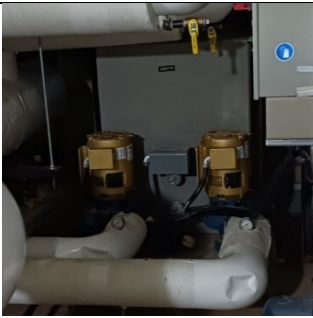
Picture 3: Condensate Receiver Unit
