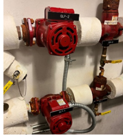
Oneida inline pumps for chilled water
