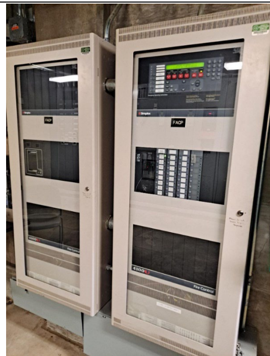
Picture 11: Fire Alarm Control Panel
