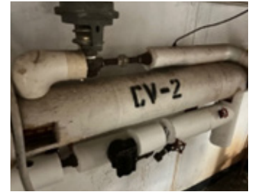
Cayuga convactor (shell and tube heat exchanger)
