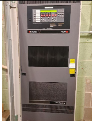
Picture 8: Fire Alarm Control Panel (FACP)
