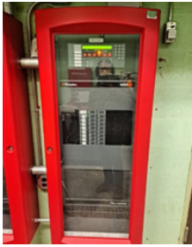
Fire alarm control panel in Hart, similar in Funnelle and Cooper
