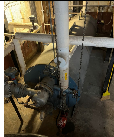
Picture 16: Domestic Hot Water Storage Tank and Steam Heat Exchanger:
