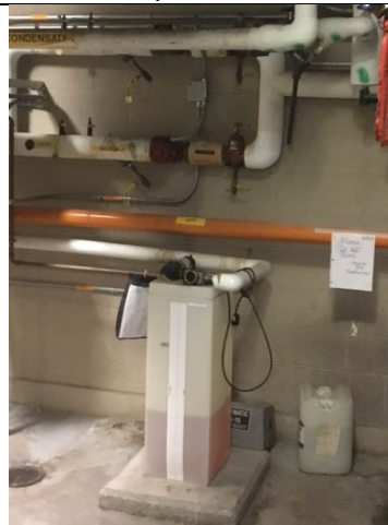
Picture 5: Glycol Feeder Tank
