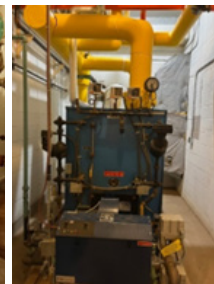
Cooper gas-fired boiler
