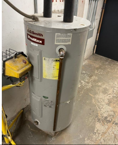
Picture 14: Electric Water Heater
