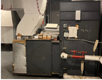
Oneida heating-ventilating unit
