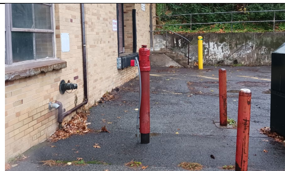
Picture 14: PIV, bollards, and FDC outside the boiler plant:
