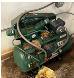
Hart Hall air compressor for pneumatic controls
