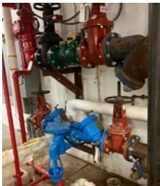
4-inch fire backflow preventer and domestic RPZ, Lakeside DH
