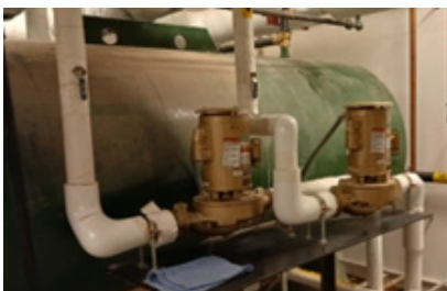
Hot water circulators in Scales
