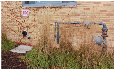
Picture 16: Gas Service with a Regulator
