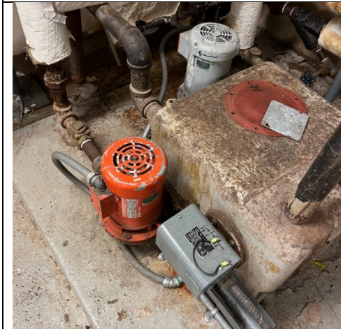
Picture 4: Condensate Receiver
