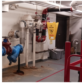
Hart incoming domestic and fire water service
