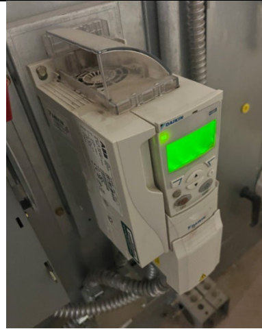
Picture 7: Supply Fan VFD
