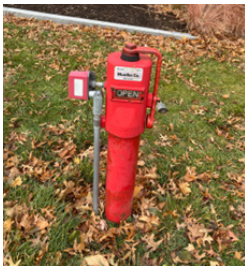
Waterbury fire service valve with tamper switch
