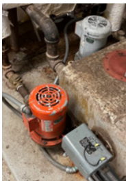
Condensate receiver in Lakeside DH
