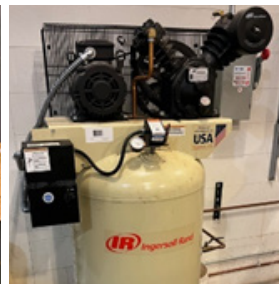
Air compressor for Cooper pneumatic controls
