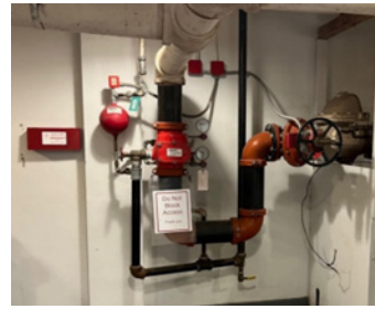
Funnelle fire protection check valve, OS&Y valve, fire alarm check valve, and spare sprinkler valve box. Sprinkler system incomplete in Funnelle, therefore inactive.
