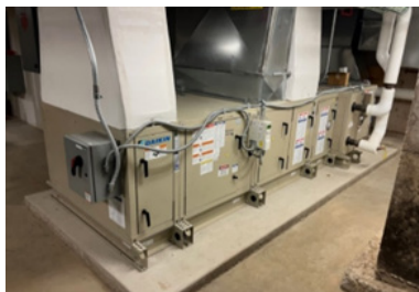
HV-1 in Waterbury. HVs serve common areas in Waterbury.
