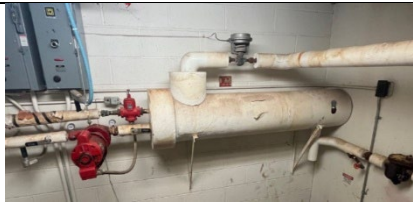
Picture 1: Heat Exchanger
