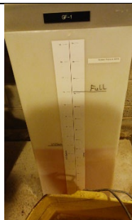
Picture 5: Glycol Feeder Tank
