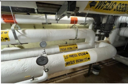
Picture 1: Pressure Reducing Valve Station
