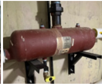
Heat exchanger in Funnelle
