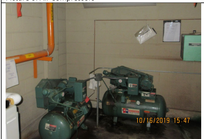
Picture 6: Air Compressors
