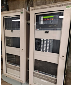
Johnson fire alarm control panel
