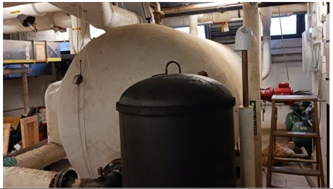
Picture 15: Domestic HW Tank
