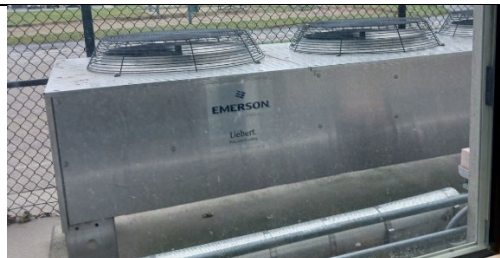
Picture 6: Fluid Cooler
