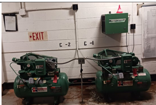
Picture 7: Air Compressors
