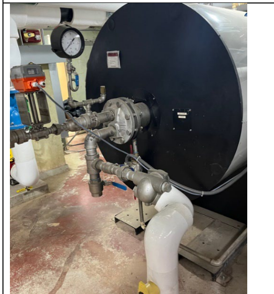
Picture 16: Domestic HW Tank
