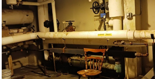
Picture 2: Steam and Condensate Lines
