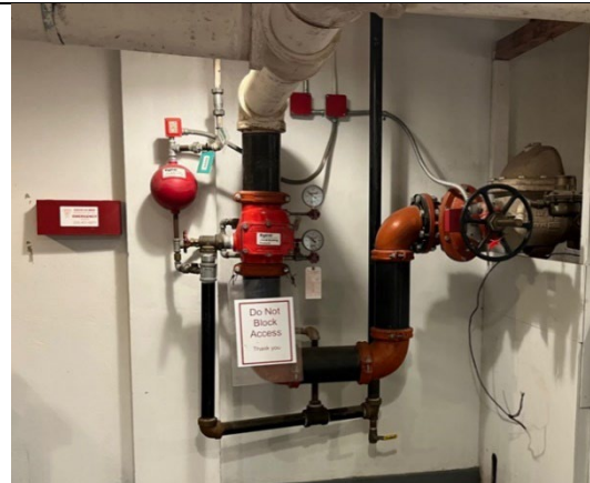
Picture 14: Detector Check Valve (gold color), OS&Y valve with tamper switch, and the fire system Alarm Check valve (red color). Spare sprinkler valve box to the left.
