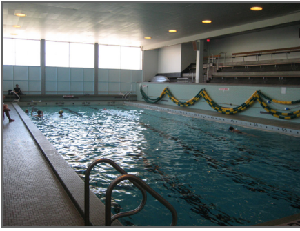
The swimming pool does not have the required ADA lift.
