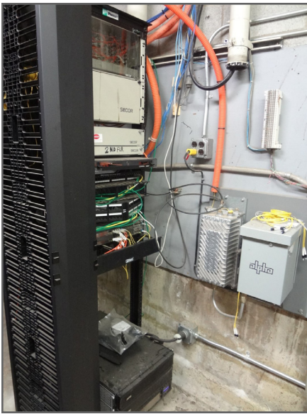
Data Rack/Telecommunications Backboard in Electric Room 12A
