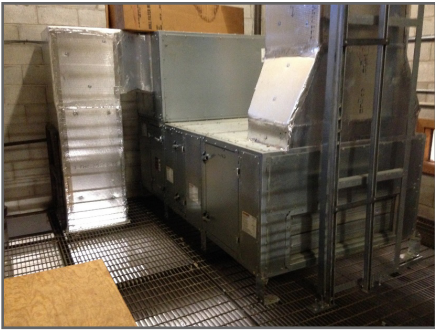
Heating and Ventilating Unit Behind Main Gymnasium
