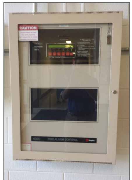
Fire Alarm Control Panel in Main Lobby
