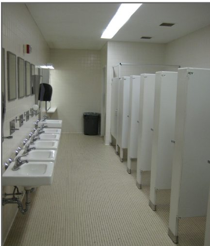
Toilet rooms have been updated, but require additional modifications to bring them into full compliance with ADA requirements.
