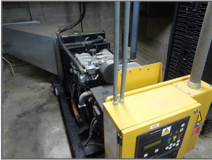
Emergency Generator in Electric Room 12A
