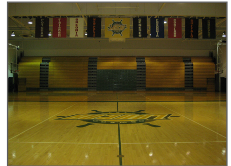
The operable partition and bleachers in the gymnasium should be replaced.
