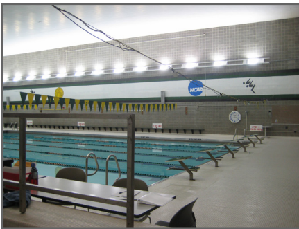
The swimming pool is in good condition.
