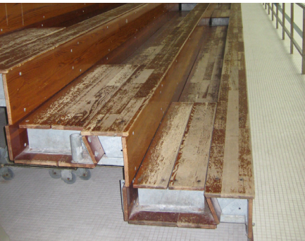
Wood bleachers in the swimming pool are in fair to poor condition.
