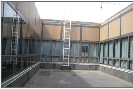
Existing single-glazed windows are in fair to poor condition.
