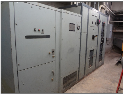
Unit Substation in Electric Room 12A
