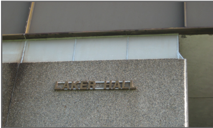
Building signage is difficult to read and should be replaced.
