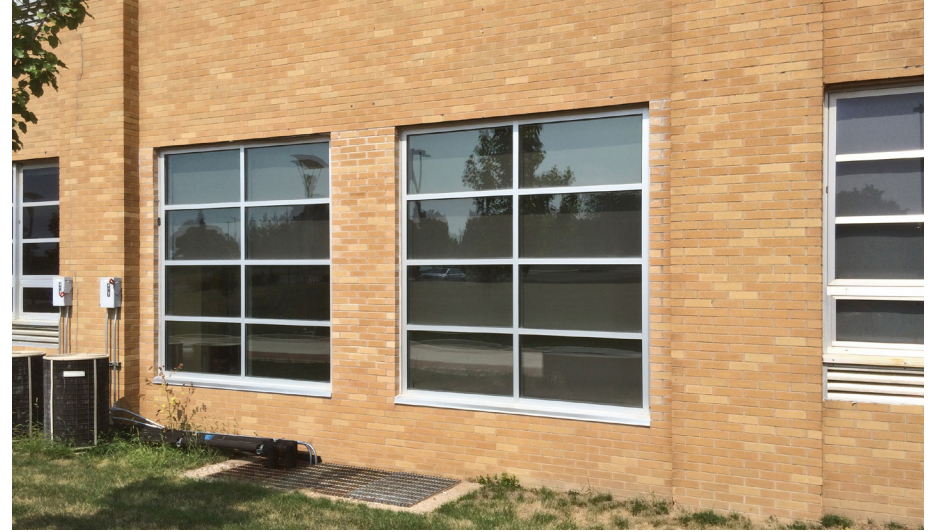
Original and 2006 windows, first floor, south façade.
