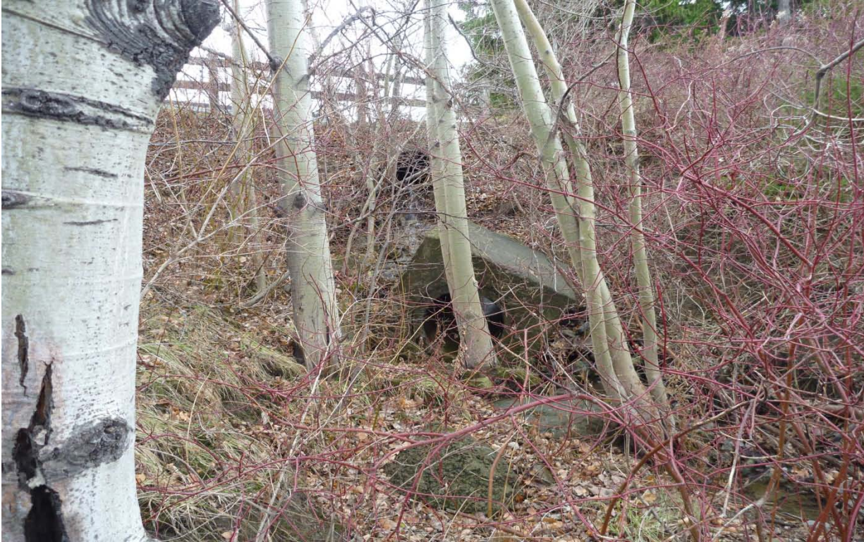
Photo 3. Looking south from shoreline at damaged central-eastern outfall. November 24, 2014
