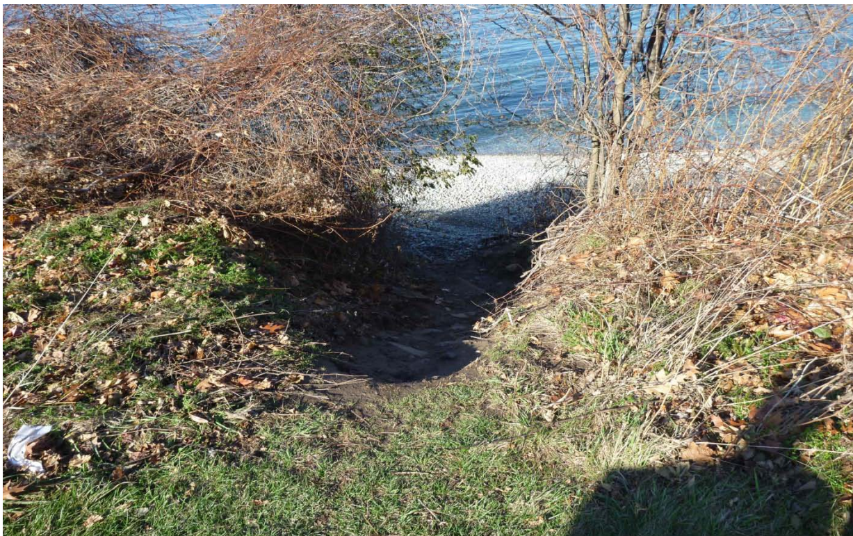
Photo 8. Erosion swale (typical) along western bank. November 24, 2014
