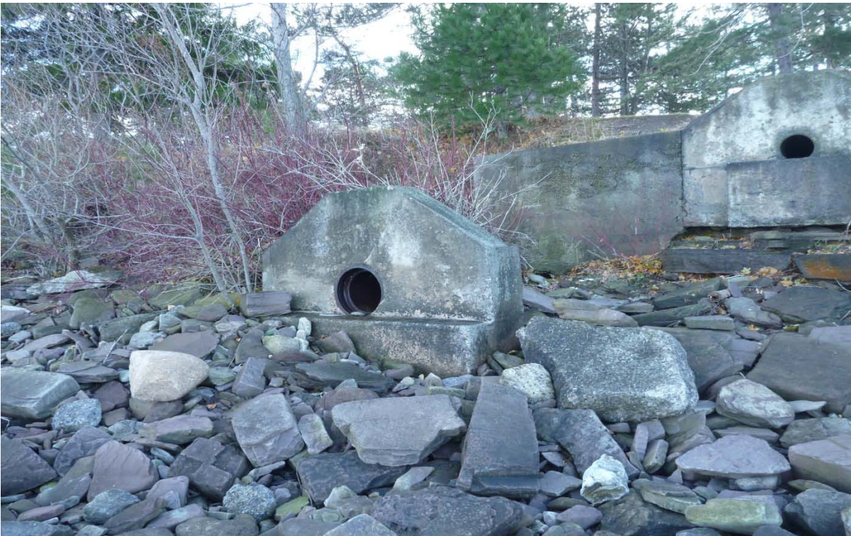
Photo 6. Looking south from shoreline at damaged western outfall. November 24, 2014
