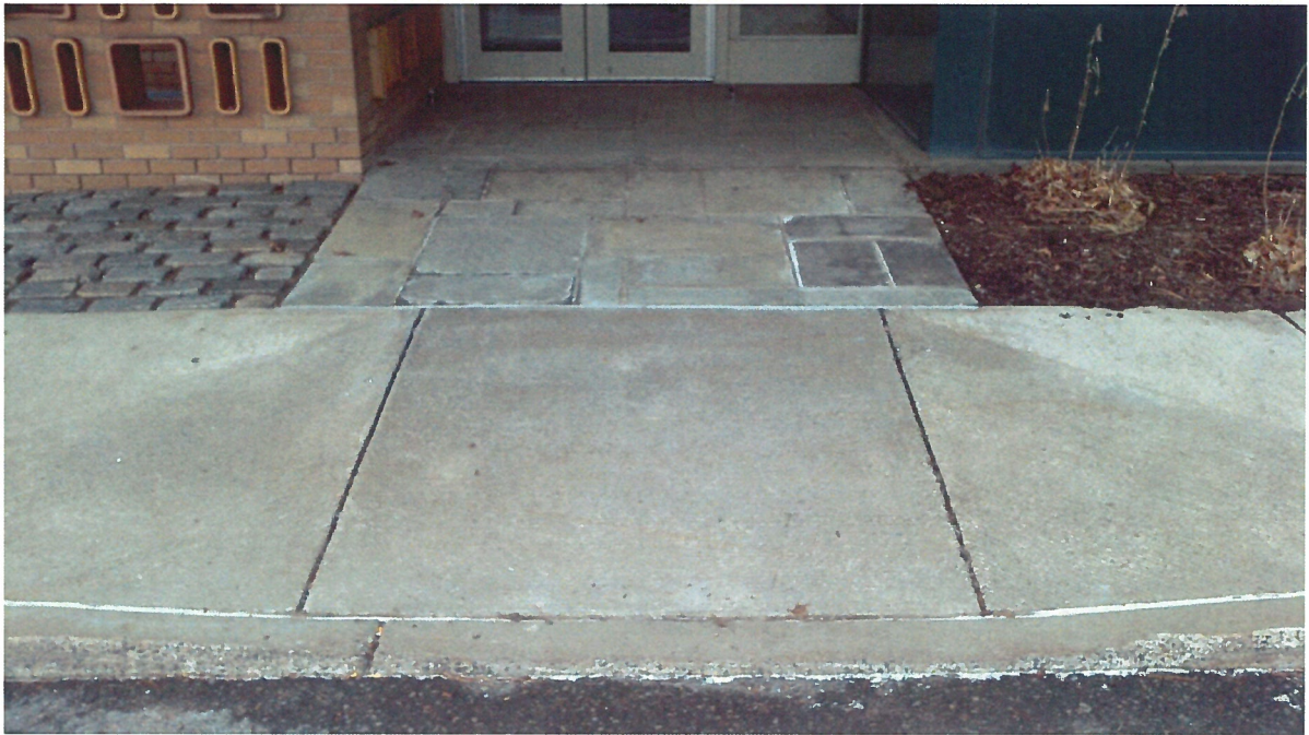
Drop-off Curb Ramp at Main Entry
