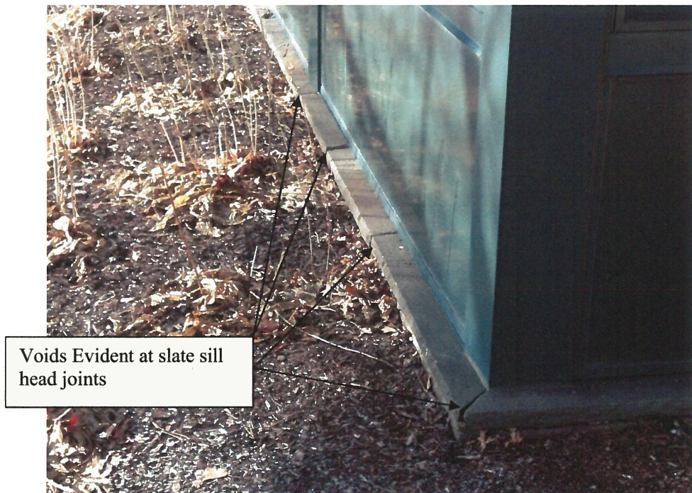
Slate Sill at Building Projection Adjacent to Front Entry
