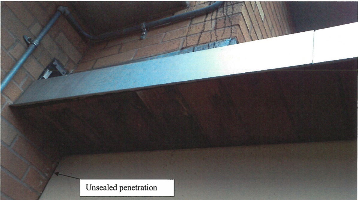
Water Damage at Front Entry Roof Soffit
