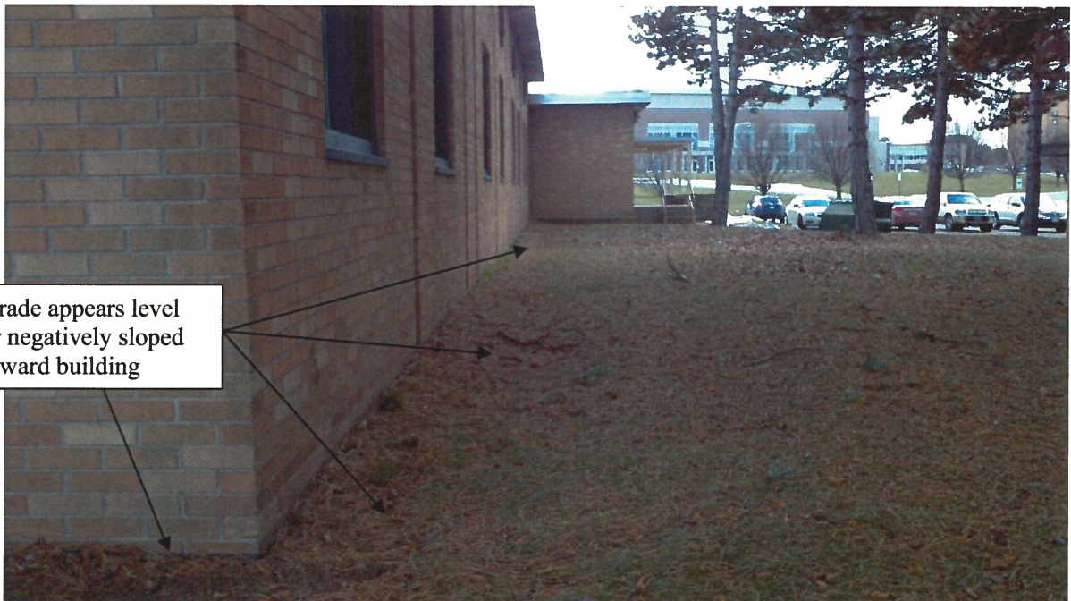
North Elevation Looking South
