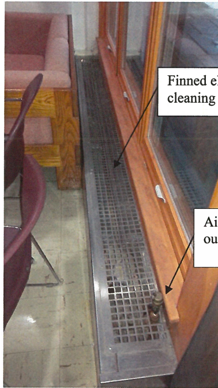
Typical Fin Tube Radiator
