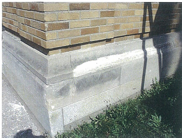
Park Hall - Limestone Base
