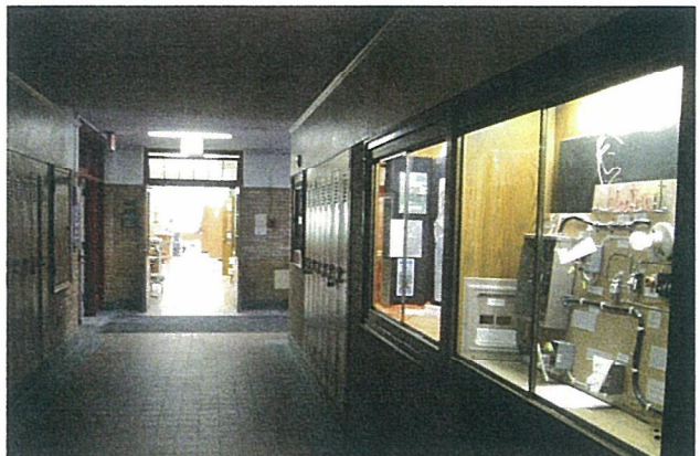
Park Hall - First Floor - Ceiling
