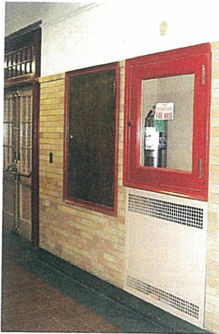
Park Hall - Corridor Walls
