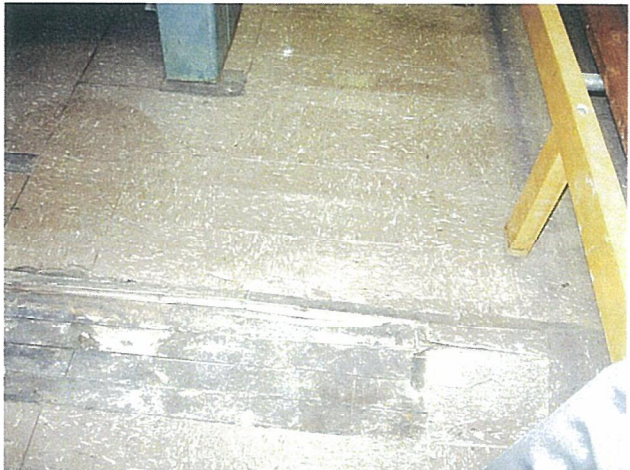
Park Hall - Room 103 - VCT flooring
