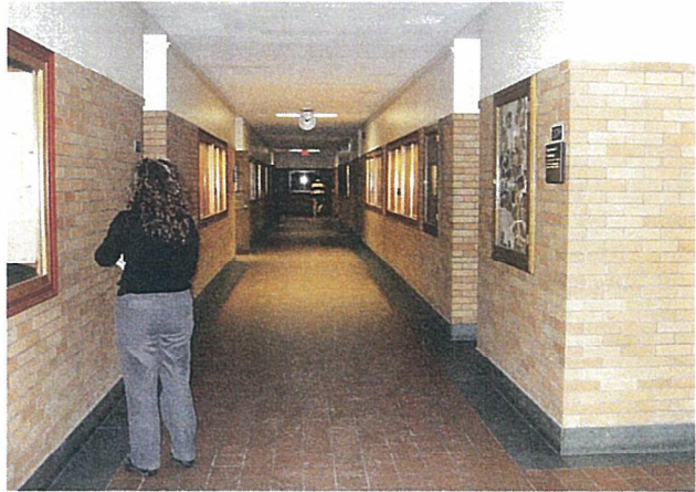
Park Hall - Second Floor Corridor
