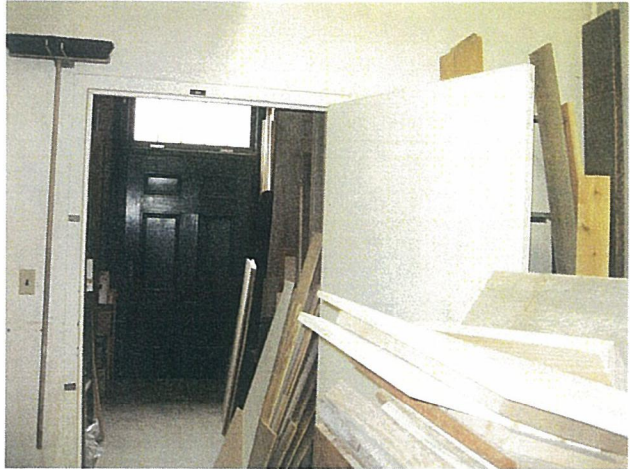
Park Hall - Room 102 - Adjacent Storage Room
