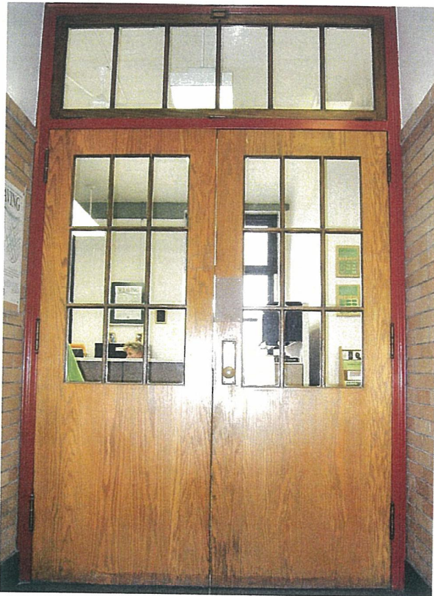
Park Hall - Third Floor Corridor Doors
