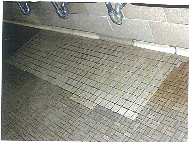
Park Hall - Suite 307 - Millwork Concealing Decommissioned HVAC Unit
