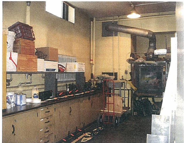
Park Hall - Room 105D - Storage
