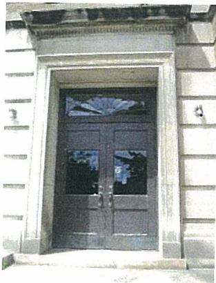
Park Hall - Exterior Doors
