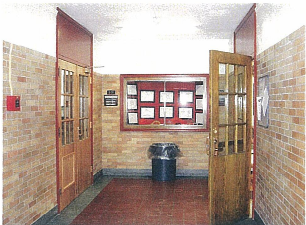
Park Hall - Second Floor Corridor - Doors
