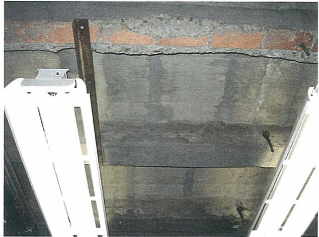
Park Hall - Basement Ceiling
