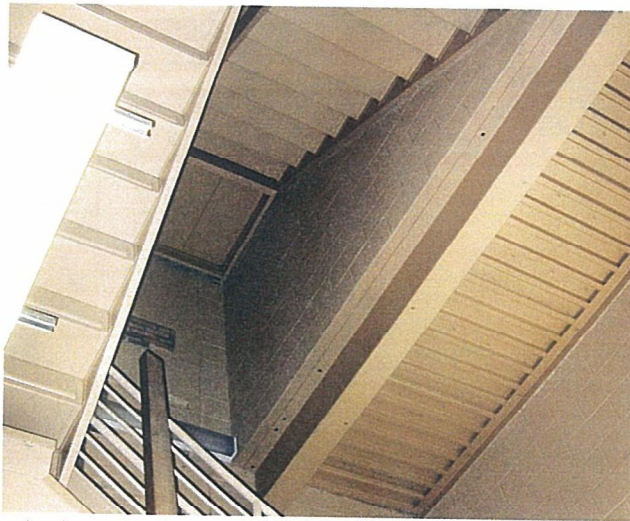
Park Hall - Room 305 - Auditorium - West Exit Stair
