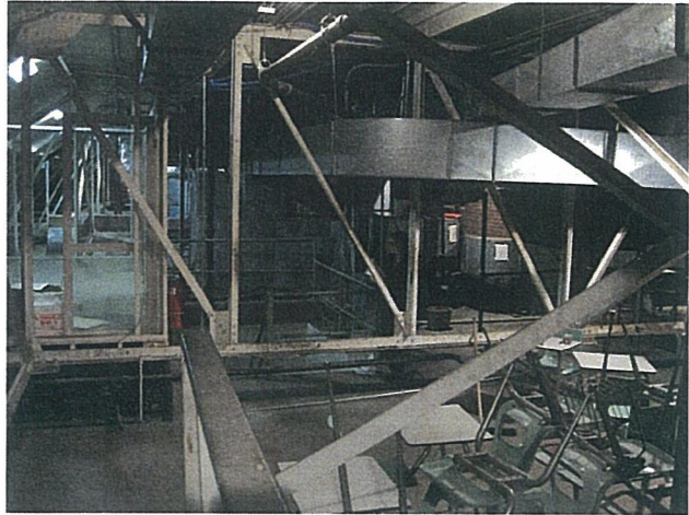
Park Hall - Attic - Truss
