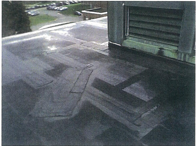
Park Hall - Roof
