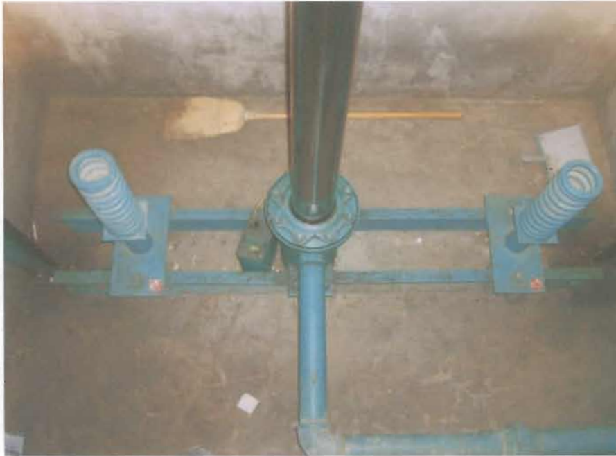
Existing Pit and Cylinder Jack Head
