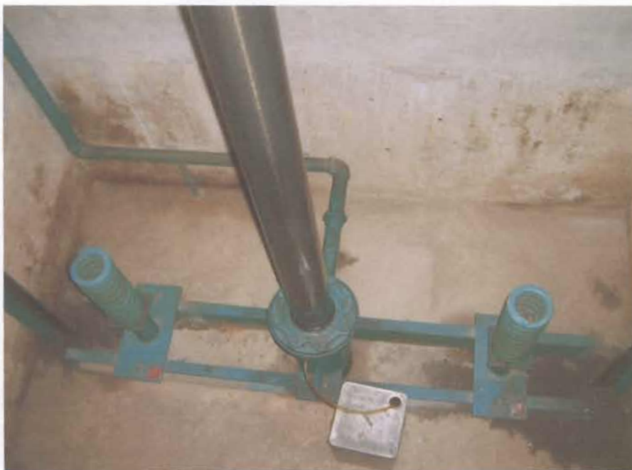
Existing Pit and Piston.
