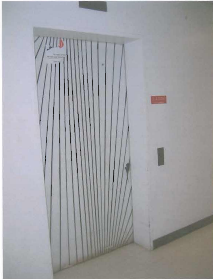
3 rd Level Lobby Landing
