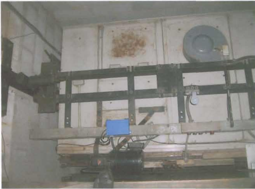
Existing Top of Car
