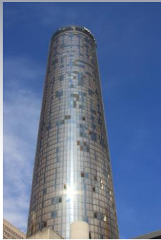
Figure 34: Atlanta skyscraper post-tornado
