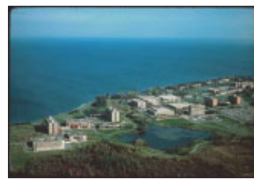
Aerial view of SUNY Oswego
