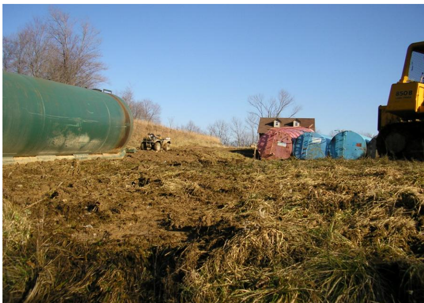
Photo: Wastewater tanks in the foreground and Mr. Boyd’s home visible in back Used with the permission of Harry Boyd
